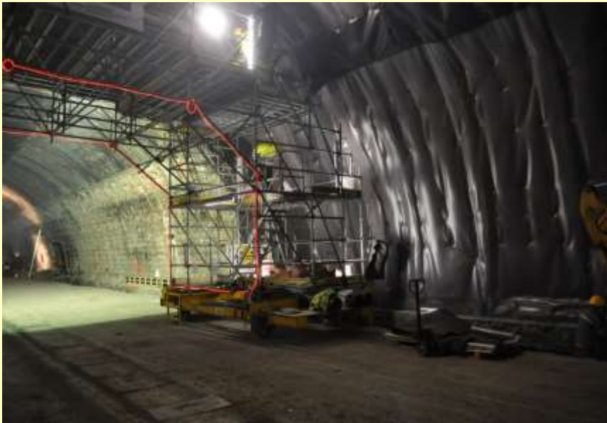
ETANCHEITE TUNNELS INTER-STATIONS
