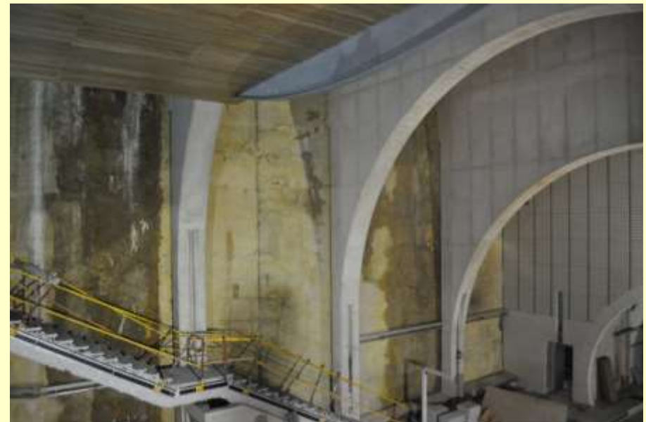
STRUCTURE RELATIVEMENT ETANCHE STATIONS - GARES
