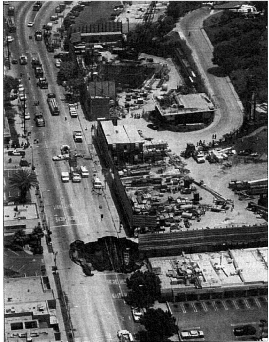
Sinkhole opened on Hollywood Boulevard over tunnel construction.
